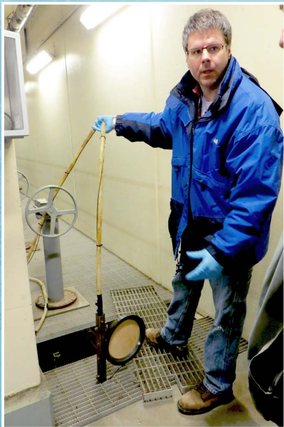
Rick Wenzel holding the 0.45 micron filter membrane for the P700 Orthophosphate Analyzer
