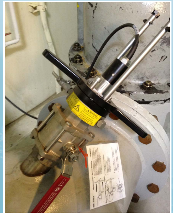
ViSolid (total suspended solids) probe in insertion mount
