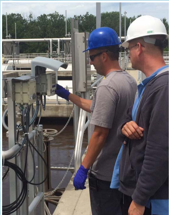
Spring Creek employees reviewing data on the YSI IQ SensorNet 2020 XT Controller
