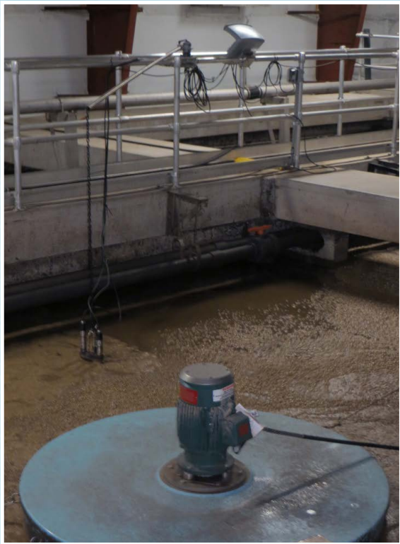
Anoxic Zone with floating mixer; TriOxmatic (dissolved oxygen), VARiON (ammonium, nitrate), and SensoLyt (pH, ORP) sensors in background
